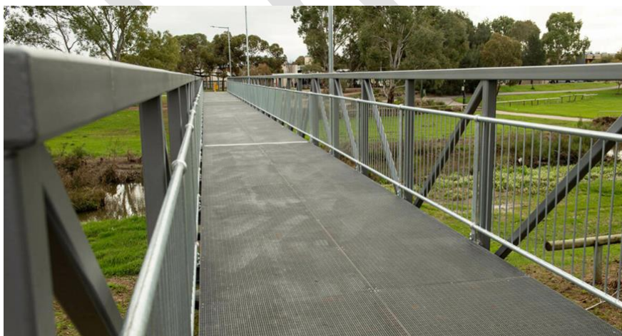
Figure 4.5 Pedestrian Footbridge at Mawson Lakes Primary School
